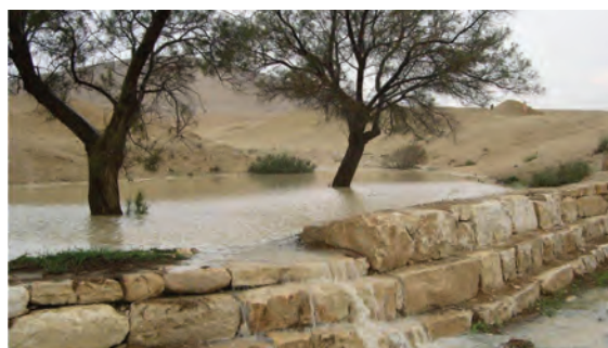
Runoff harvesting by damming streambeds.
